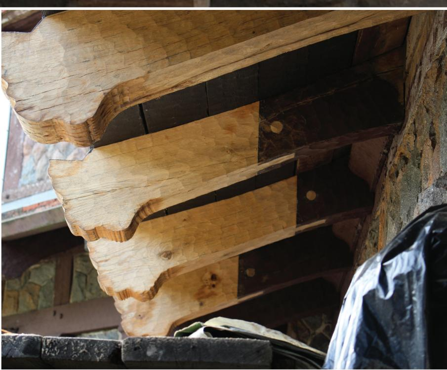
above | A pergola post gets a new section of white oak to replace a rotted area. The original is joined with the new and secured with a dowel, 2017.
