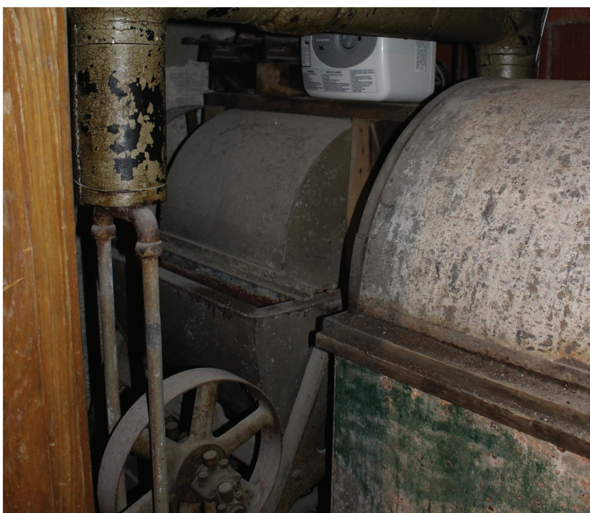
The Castle's refrigeration motor and brine tank, before restoration, 2017.
