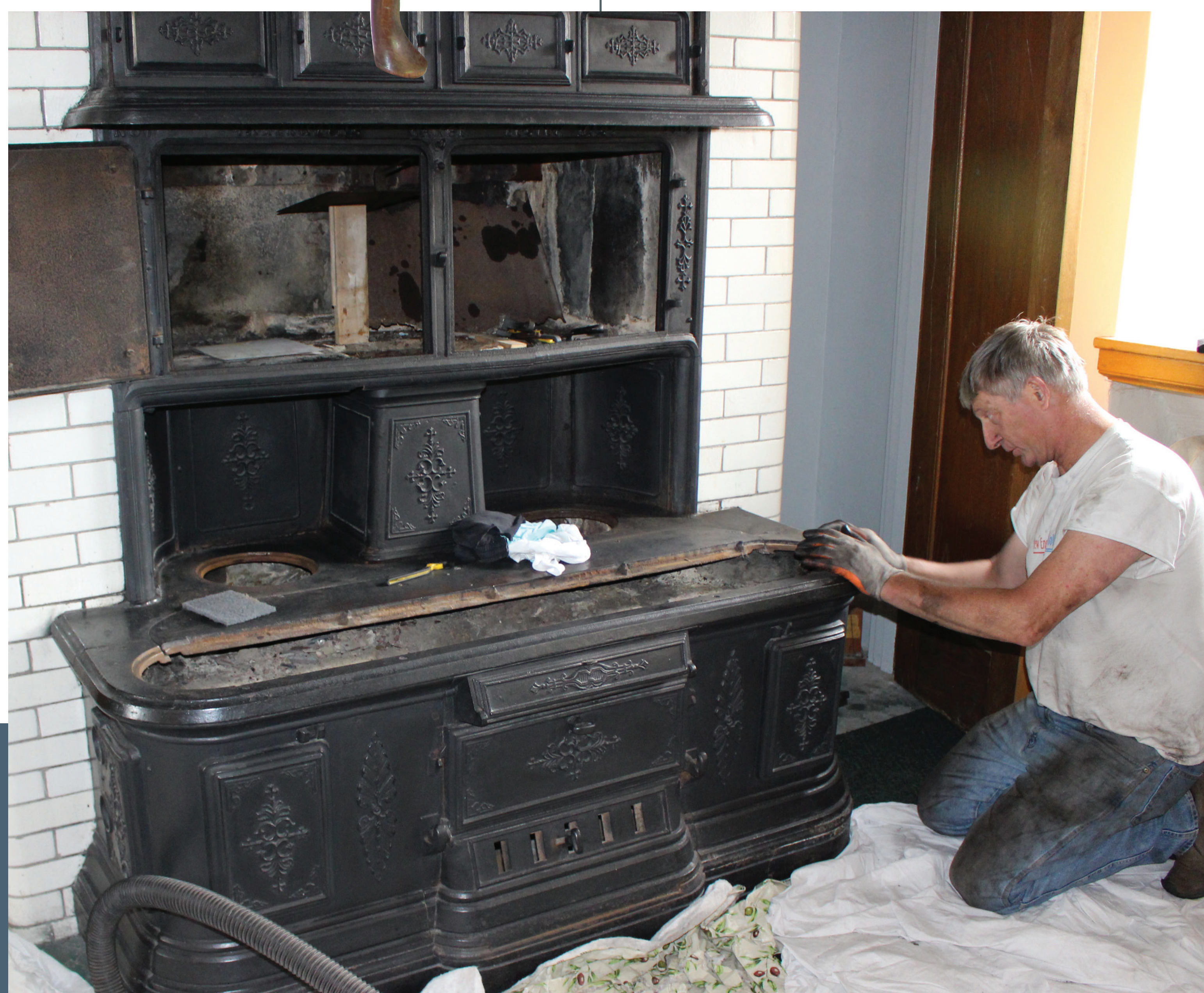
The Castle's kitchen range gets a thorough cleaning and protective coating by Graham Barber of Graham the Stove Man – Woodstove Repair and Restoration, 2017.
